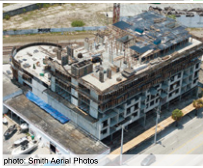
photo: Smith Aerial Photos
